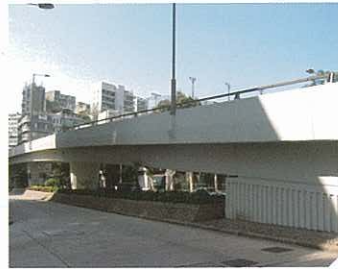
Highway Department in Hong Kong
